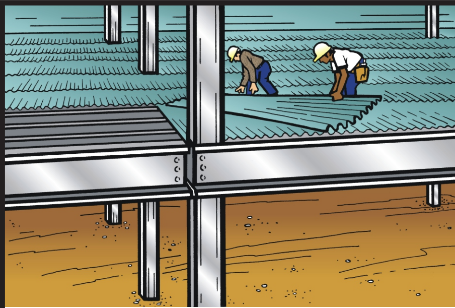
Figure 1 - INCORRECT No fall arrest system or guardrails in use
